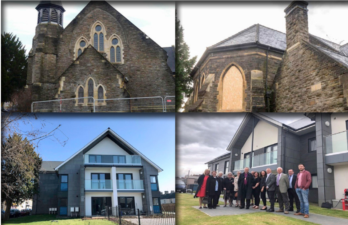
▲ St Matthews Church, Newport. Before the work started, after work was finished, and a visit from the Archbishop of Wales.
