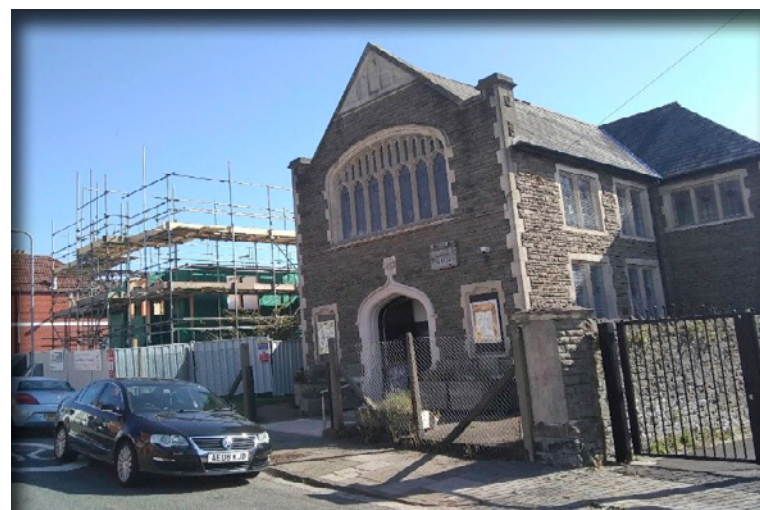
▲ Pentyrch Street Baptist Church, Cathays, Cardiff.
