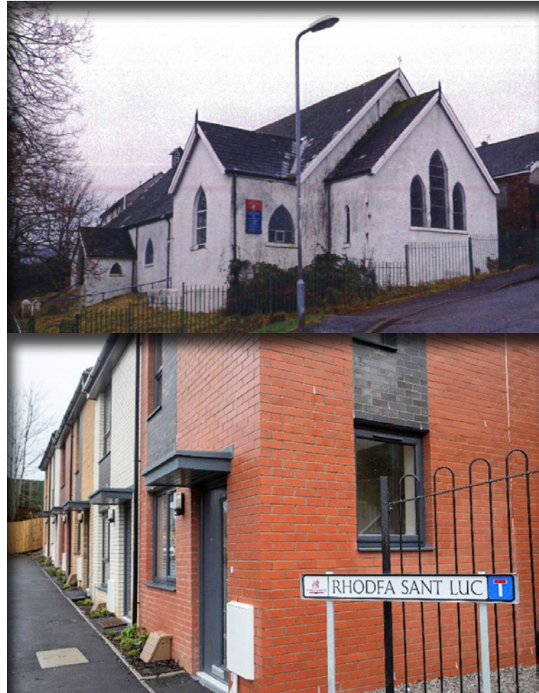
▲ New houses built on the St Lukes Church in Porth.
